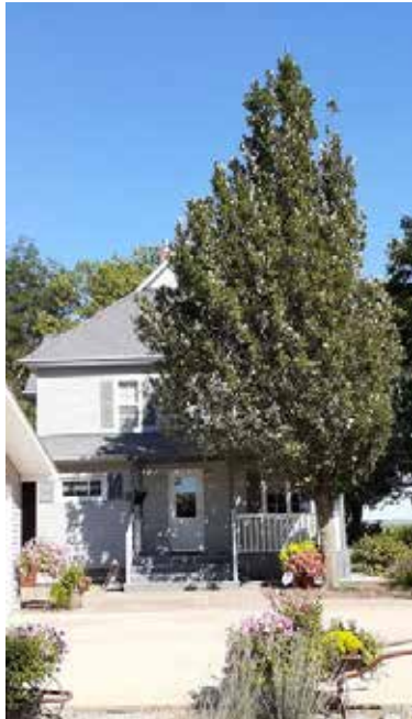
Exterior of Home
